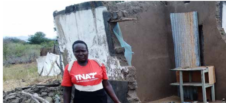
Severina's shuttered shelter after the heavy rains in March 2018
