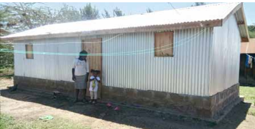
Leah's completed house
