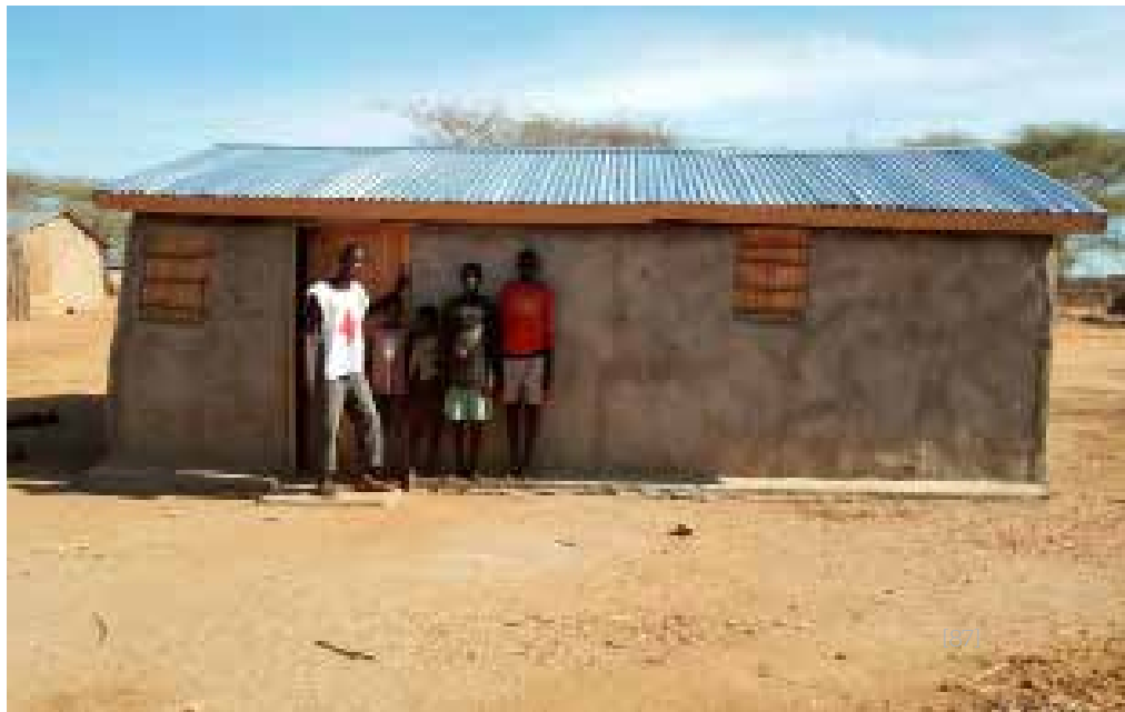
PICTURE 2: LOBEI, HIS SIBLING AND A KRCS VOLUNTEER OUTSIDE THEIR FINISHED HOUSE
